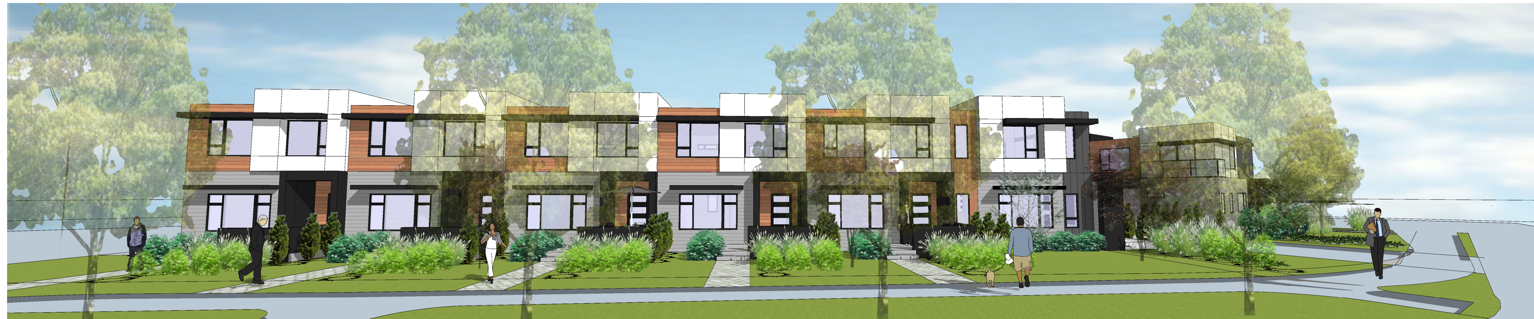
STREET SCAPE ALONG GODFREY FACING EAST
